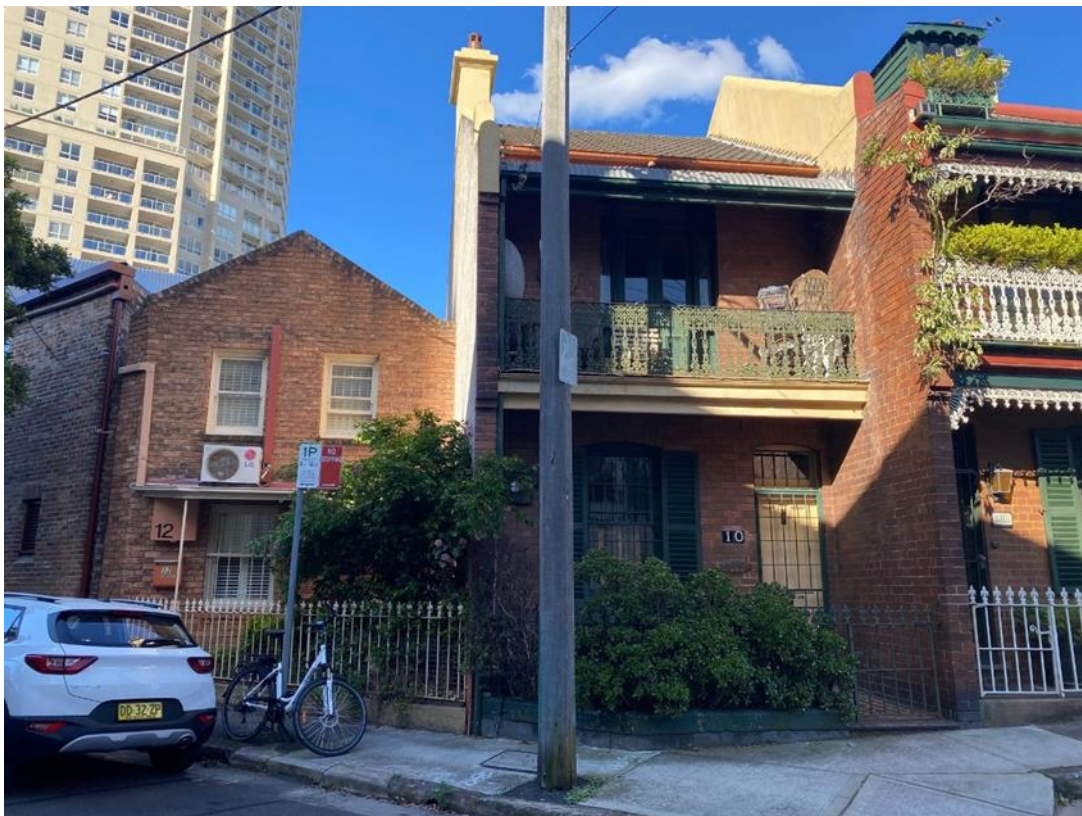
Figure 6: 12 Nimrod Street and adjoining development to the south-east, viewed from the south-west
