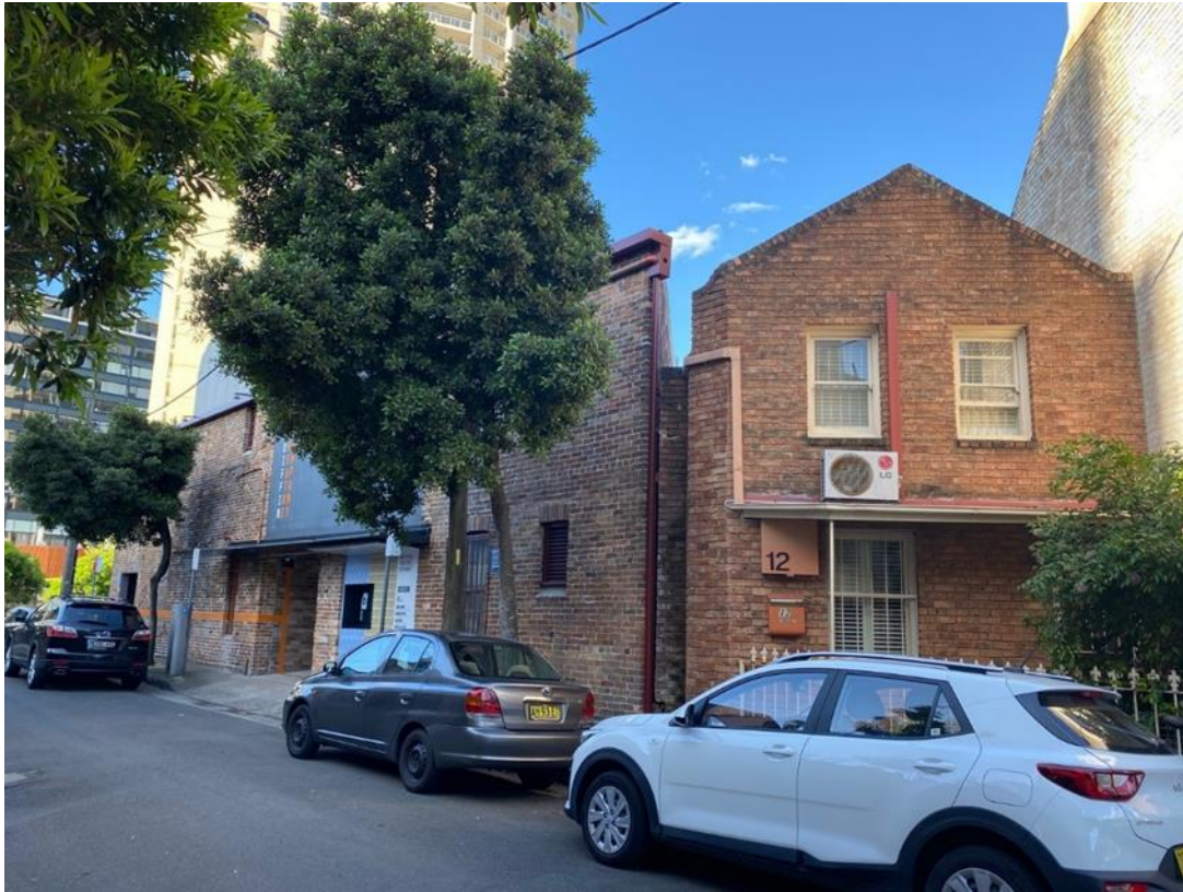
Figure 5: 10 and 12 Nimrod Street viewed from the south-west
